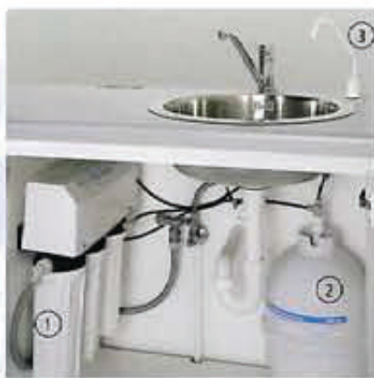
MELAdem ® 47 (1) installed in a sub cabinet with water tank (2) and additional tap (3).
